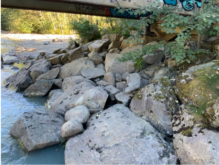
Right Bank Abutment when facing downstream
