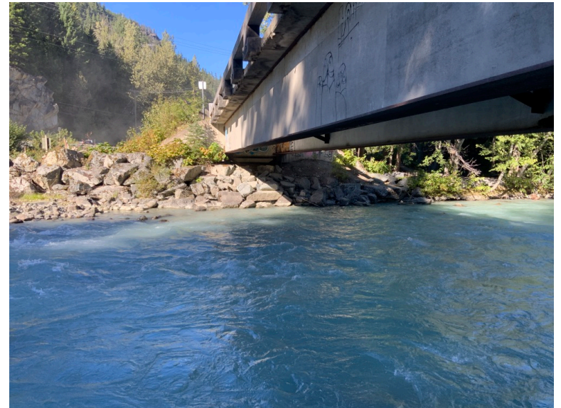
Left Bank Abutment when facing downstream
